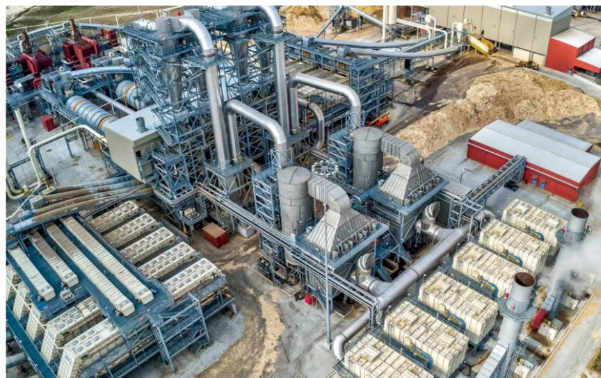
Application of Part.X PV venturi scrubbers, Part.X PW wet ESPs and Oxi.X RC RTOs in the engineered wood products industry.
